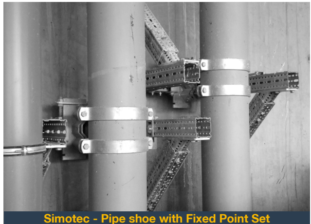
Simotec - Pipe shoe with Fixed Point Set
